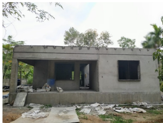
Fig.4.3 ferrocement residential building
