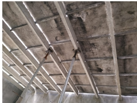
Fig. 1.2 ferrocement roof tops.
