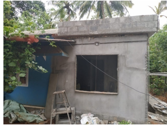
Fig.4.1.ferrocement expansion work
