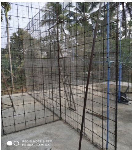
Fig. 1.1 frame work of wall construction.
